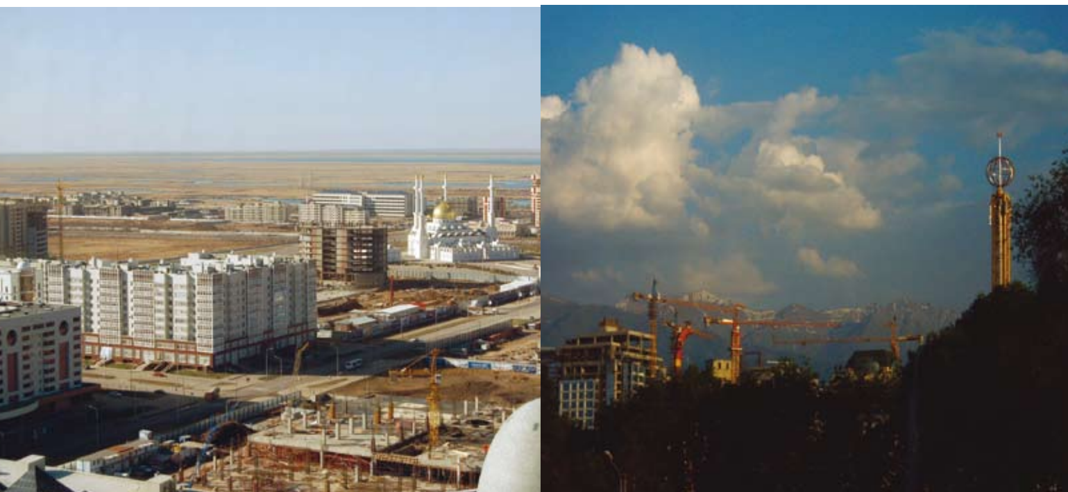
Construction boom in the two major cities: Left, the new capital Astana in the northern steppeland. Right, the southern "capital" and financial center Almaty at the bottom of the Tien Shan Mountains.
